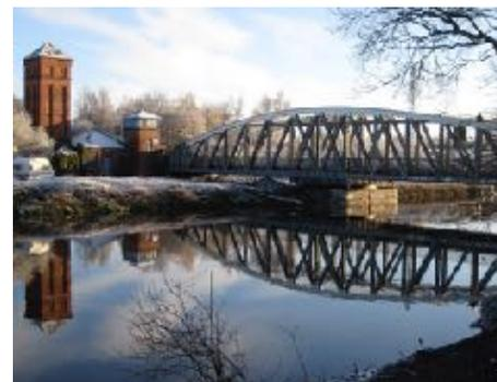
**Moore Lane Swing Bridge** - One of seven on the canal, all hydraulically powered, the original steam engines have long been replaced by more modern machines. The structure, when new, weighed 700 tons, it uses 64 roller bearings with a turning diameter of 28 feet.
